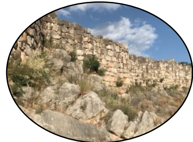
F. Southwestern Fortification Wall, upper citadel (view south)
